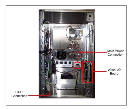
Figure 5. C-Start Interior Connections
